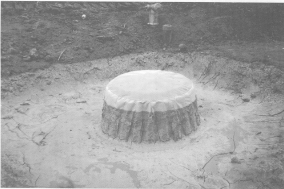
Figure 6-21.7 - Alternative Inlet Sediment Trap
