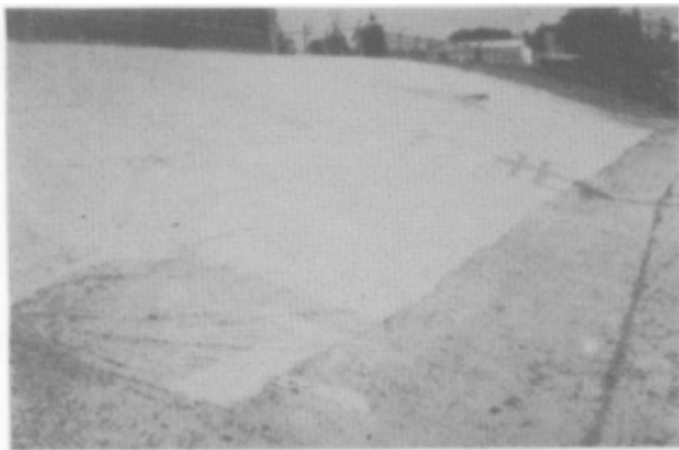
Figure 2-9. - Jute matting can assist in rapid establishment of vegetation.
