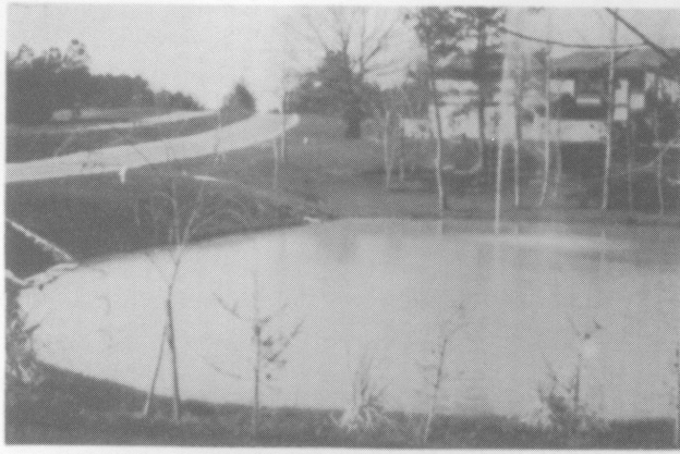
Figure 2-13. - A temporary sediment basin converted to a permanent pond enhances landscape.
