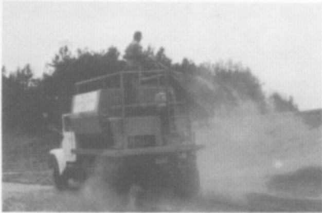
Figure 2-8. - Hydroseeding equipment can efficiently and quickly establish disturbed areas.
