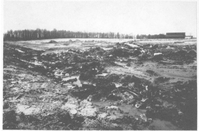
Figure 1-1. - Erosion on this construction site was the result of poor planning.
