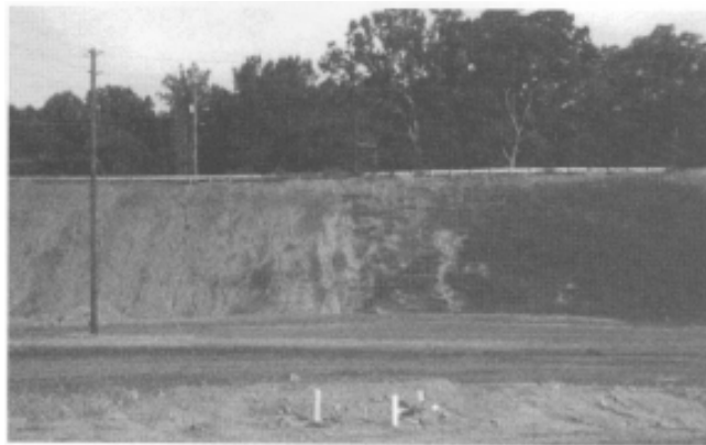
Figure 6-8.1. Hydroseeded Slope with and without Polyacrylamide Application
