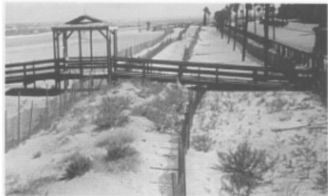
Figure 6-2.1 - Sand Fence and Native Plants
