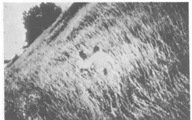
Figure 2-7. - Vegetation on this road bank will reduce erosion to a minimum.
